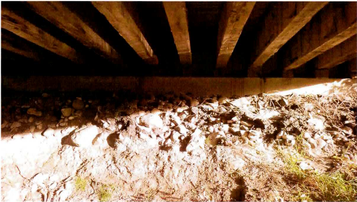
SU1, North abutment
