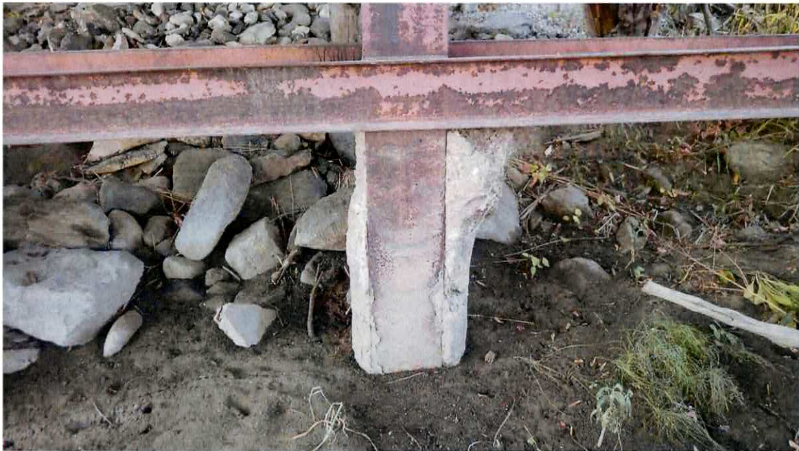
SU4 pile at groundline. NOTE: Concrete has been cast around the pile bases. (1)
