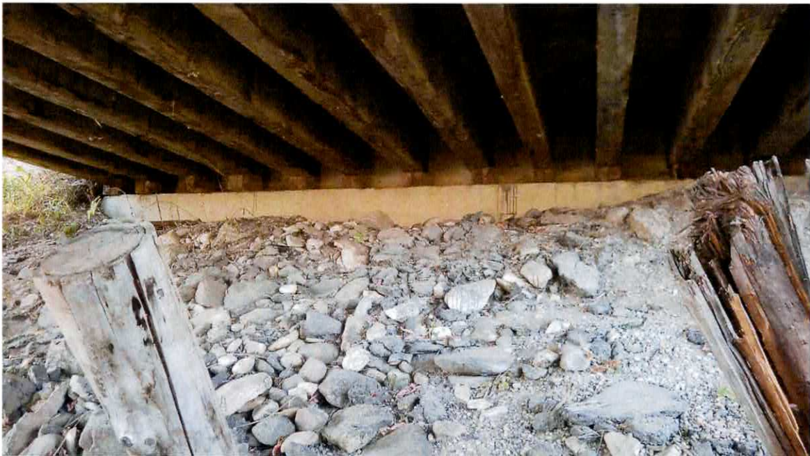
SU5, South abutment. NOTE: Spacer blocks under girders
