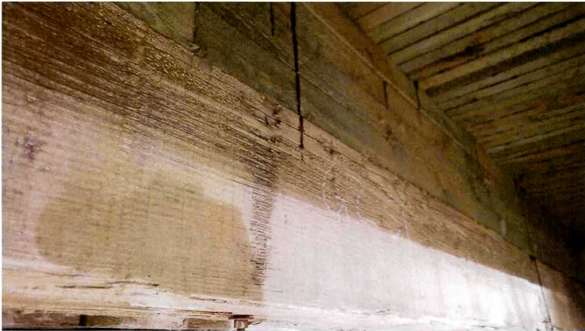
G6, span 1. NOTE: Girder is only half height and top half is constructed of other timbers
