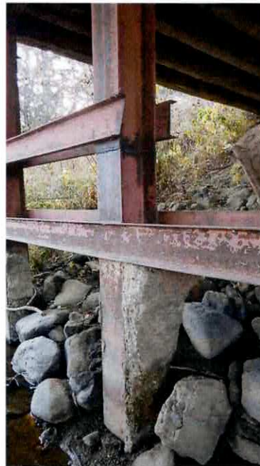
SU4 pile at groundline. NOTE: Concrete has been cast around the pile bases. (2)
