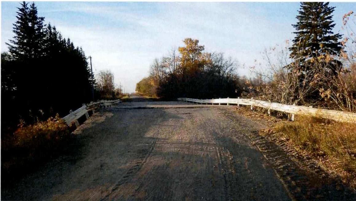
Roadway, looking South
