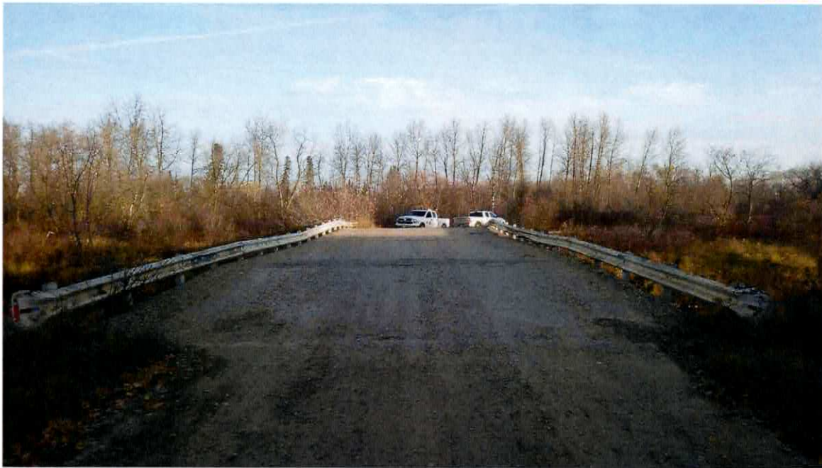
Roadway, looking North
